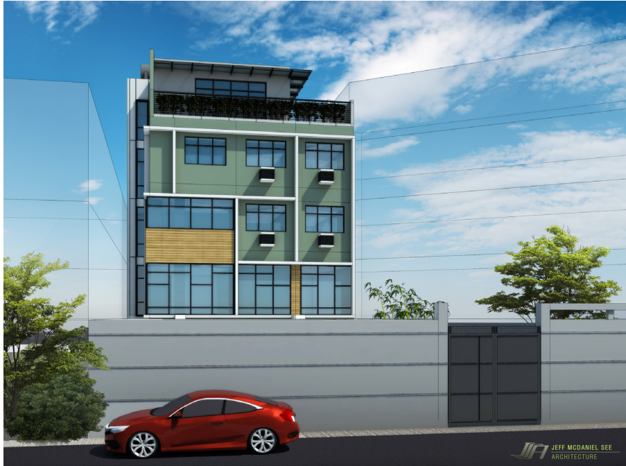
4-storey apartment residence Grace Park, Caloocan
