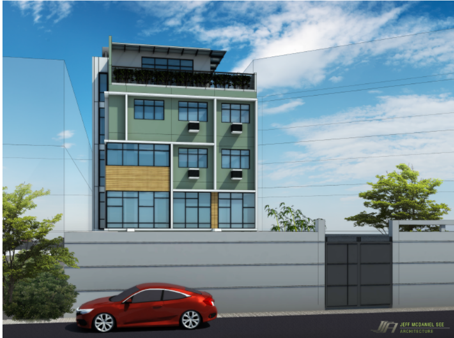
4-storey apartment residence Grace Park, Caloocan
